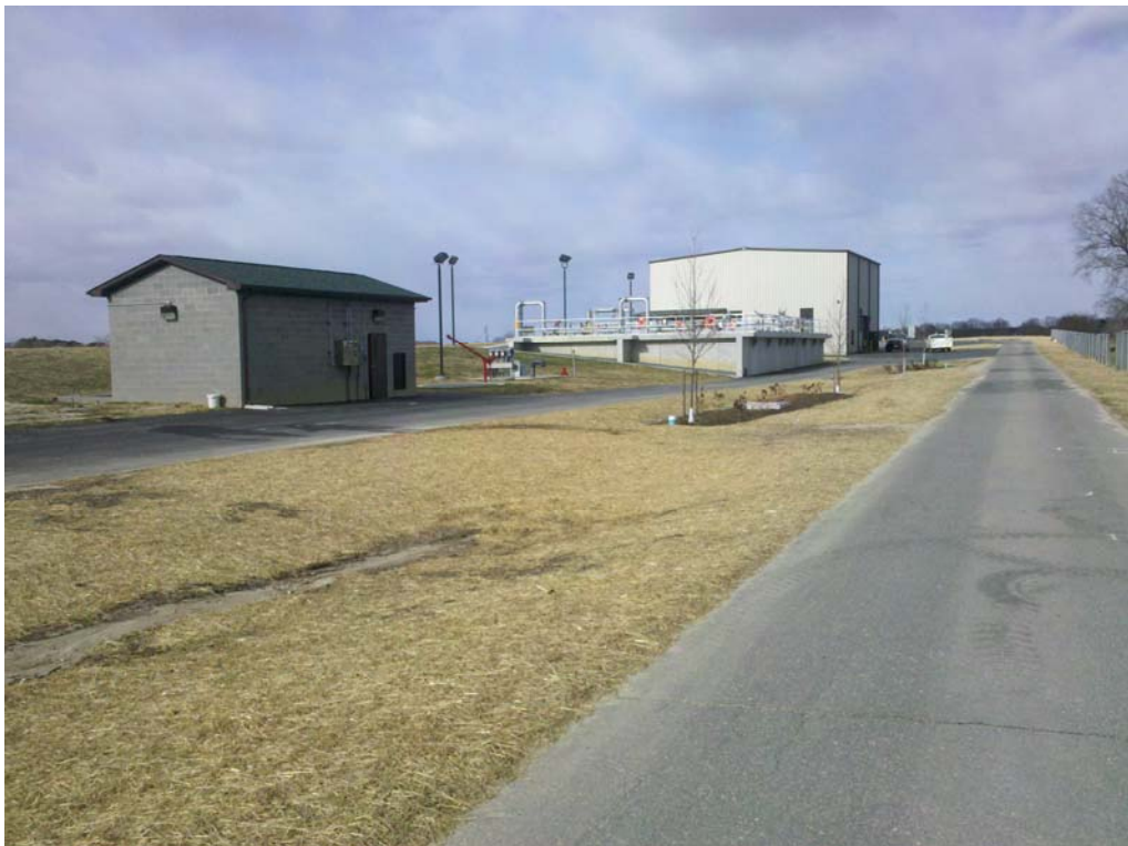
Completed WWTP - Screen Building, Aeration Basins and Operations Building Pictured
