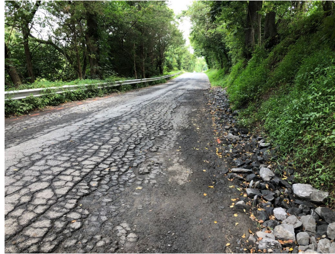
Base Failure
