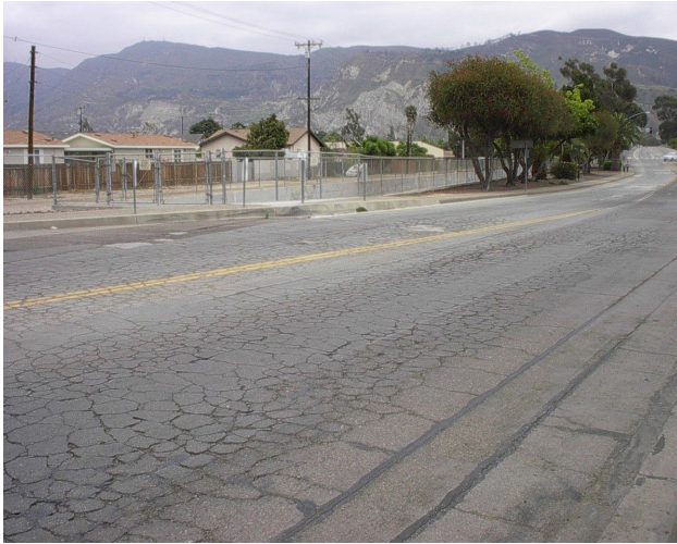
Fatigue Cracking – High With High Traffic Volume
