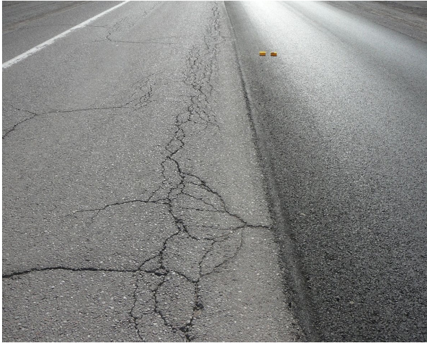
Fatigue, Longitudinal & Transverse Cracking – Moderate
