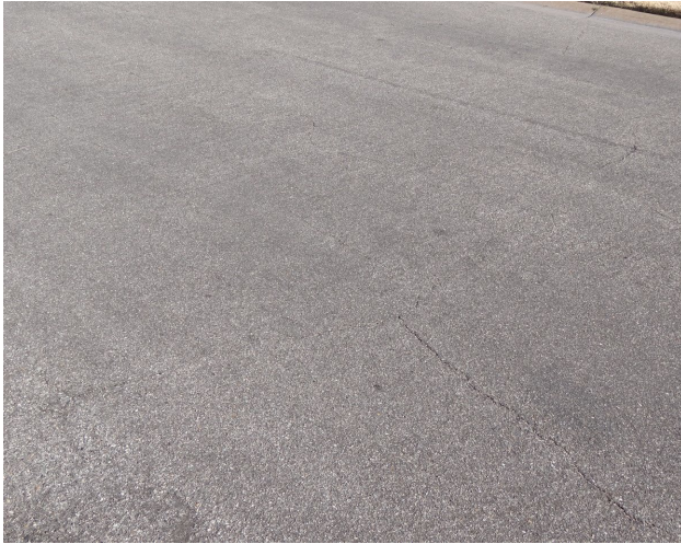
Fatigue Cracking – Low
