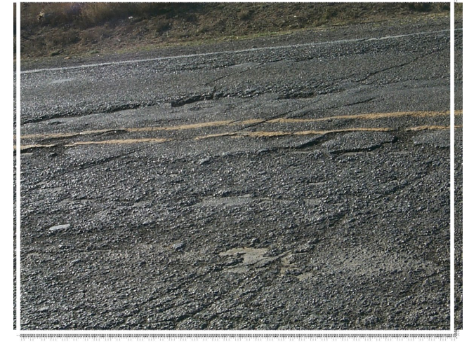
Oxidation and Raveling – High
