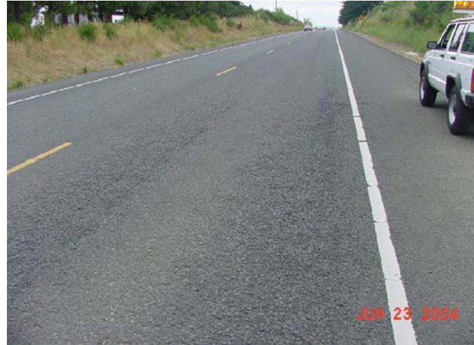
Oxidation and Raveling – Moderate
