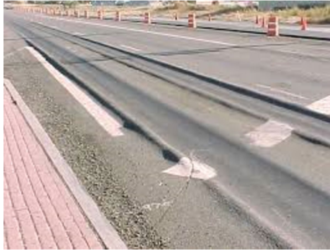
Rutting – High With High Traffic Volume
