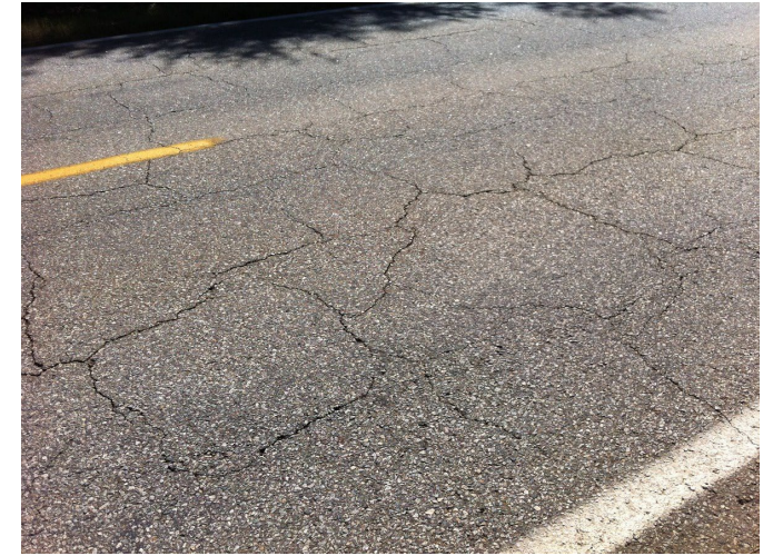
Longitudinal & Transverse Cracking Moderate
