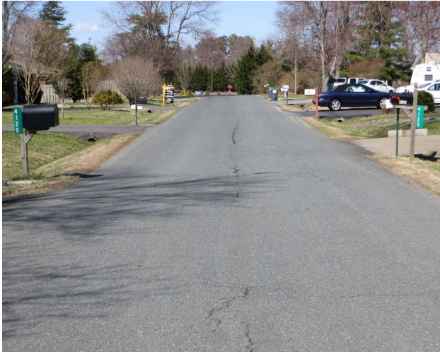
Fatigue Cracking – Low
