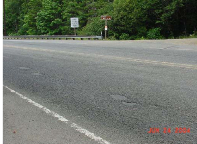
Oxidation and Raveling – High
