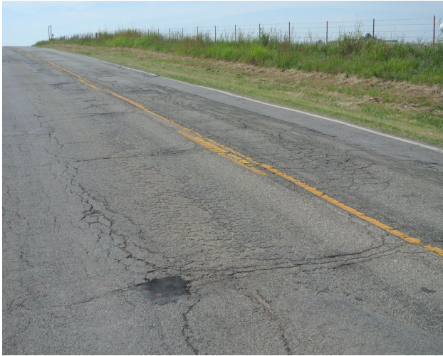
Fatigue Cracking – High Potholes
