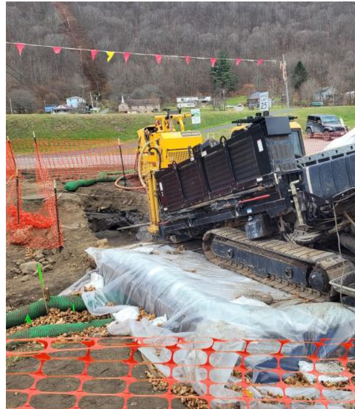
HDD boring photo courtesy of Leonard Cage, MDE Compliance Program.
