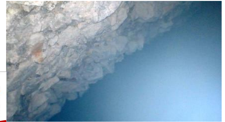
Underside of approach slab with void below
